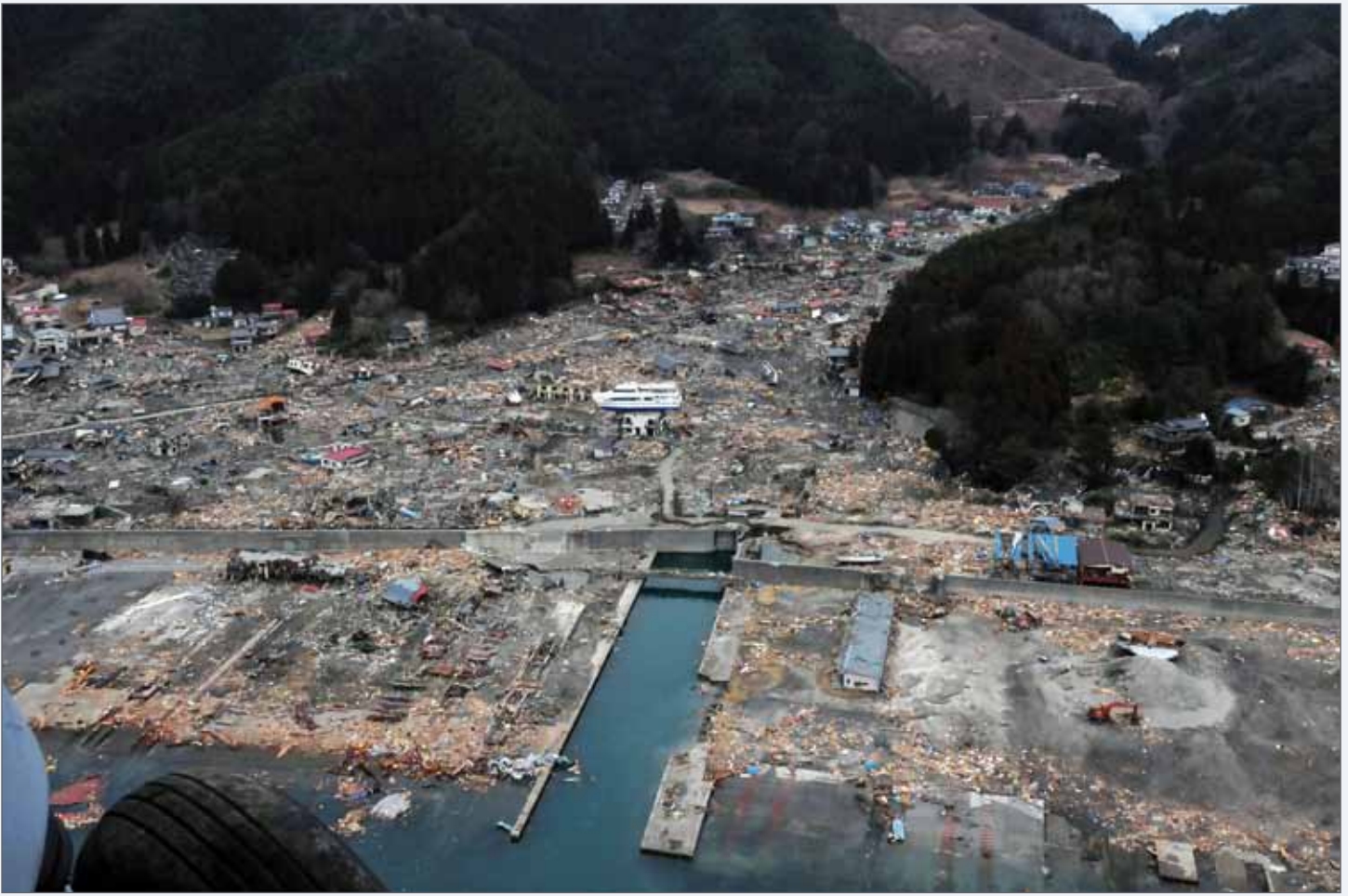
An aerial view of damage to Wakuya, Japan after a 9.0 magnitude earthquake and subsequent tsunami devastated the area in northern Japan. Ships and aircraft from the Ronald Reagan Carrier Strike Group conducted search and rescue operations and re-supply missions in support of Operation Tomodachi throughout northern Japan.
